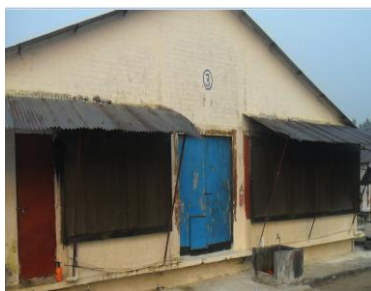
Fig 2: In front of Shed with Evaporating Cooling System.
