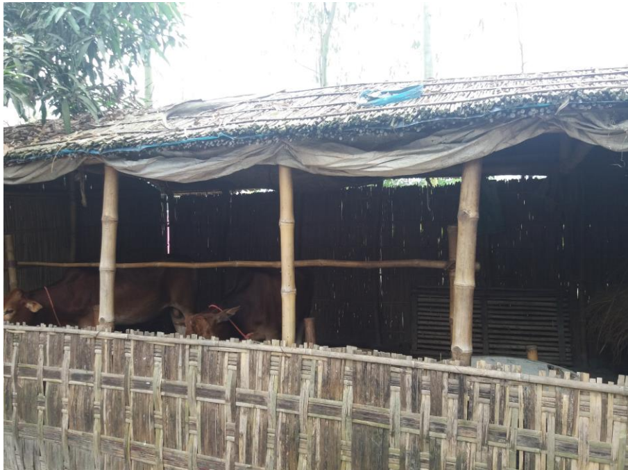
(b) Showing Roof made by Jute stick
