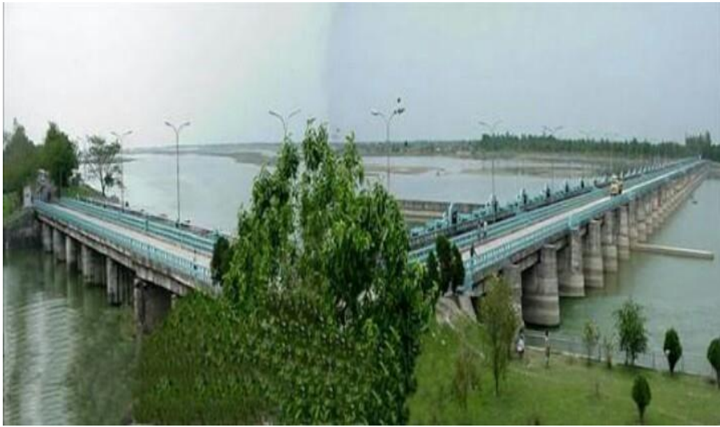
Figure : 3.11, Teesta Barrage
