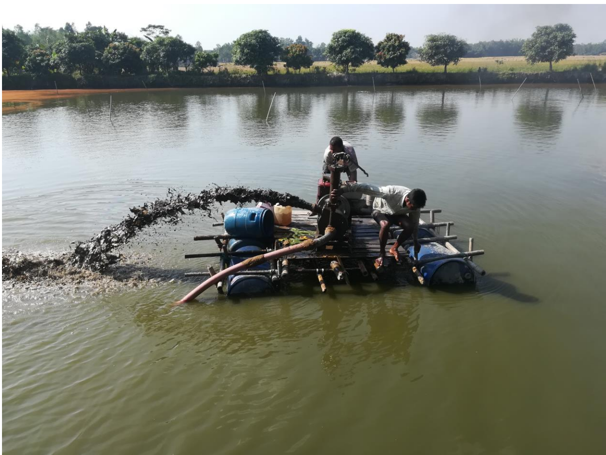
Figure 3.14: Field trial of the Sludge remover
