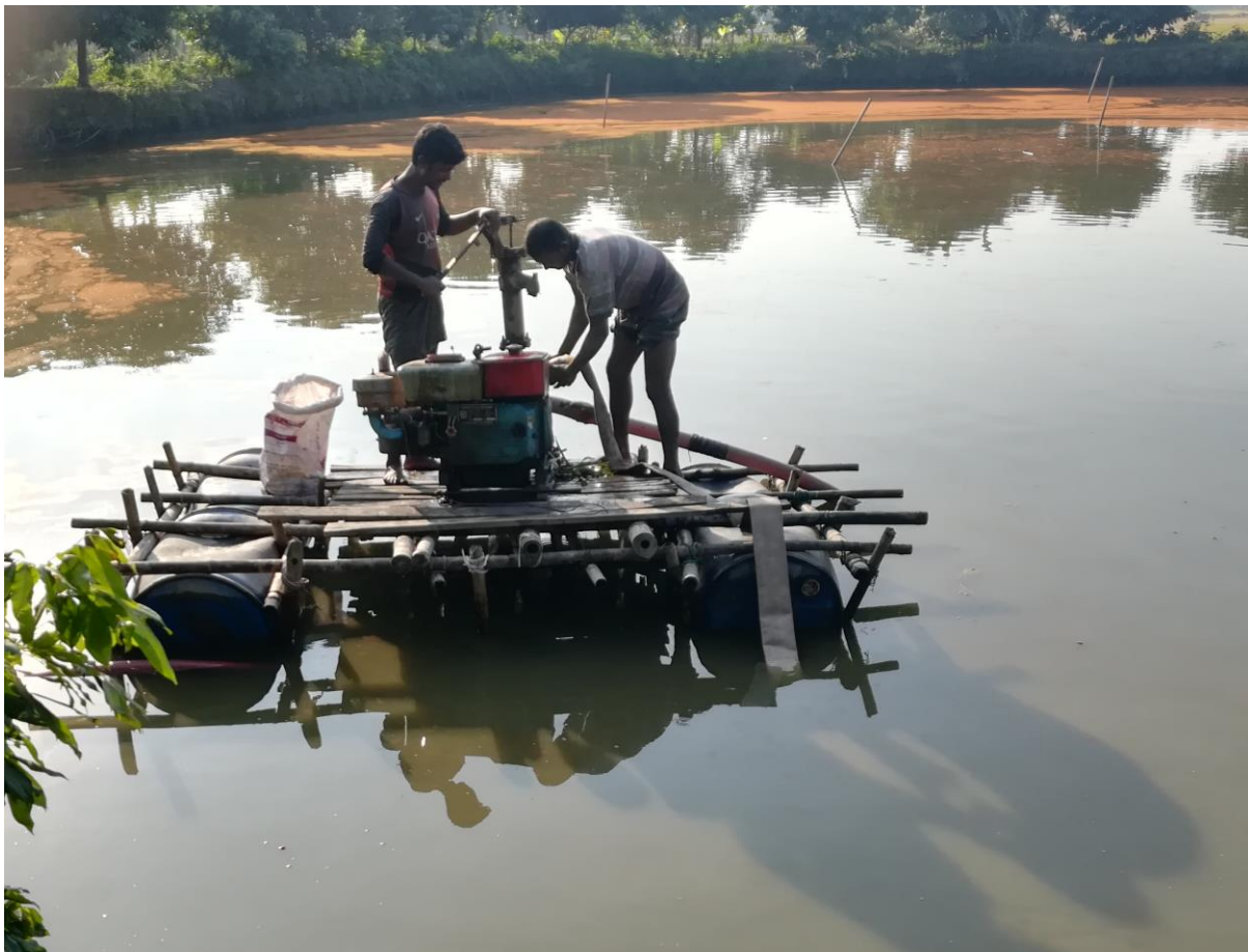
Figure 3.13: Operation of the Sludge remover
