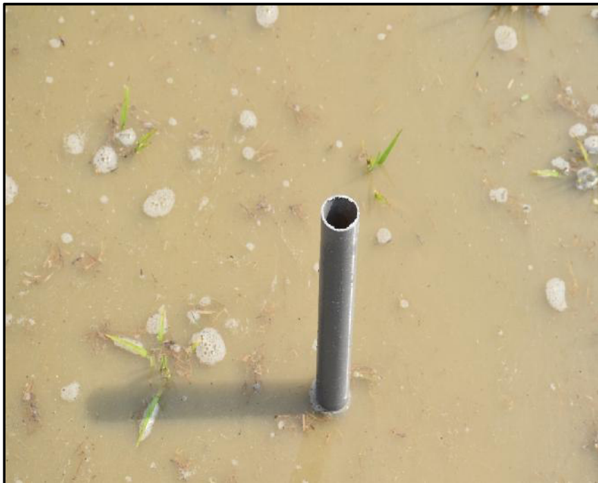
Figure 3-5: Installation of PVC Pipe for Measuring Seepage and Percolation Loss
